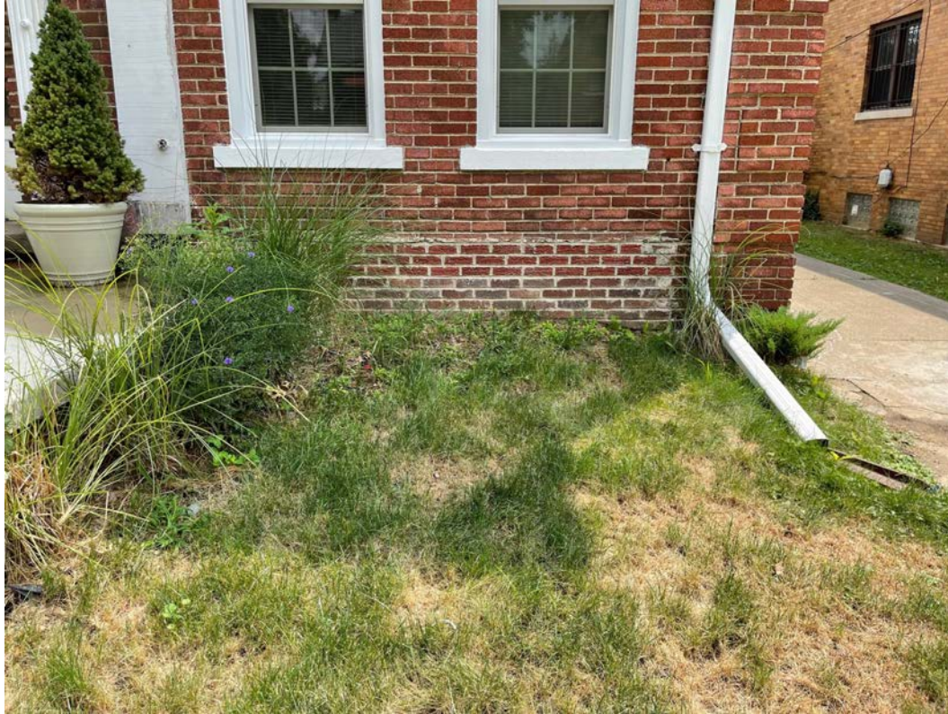
PLANTER LOCATION - WEST SIDE
