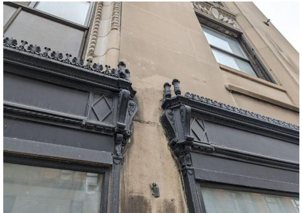
*Site Photo 4, by Staff March 27, 2024: (west elevation) showing cast iron header detail over storefront, and newer storefront window units fitted carefully into the original frames.*
