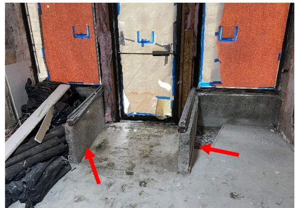
Site Photo 3, by Staff April 2, 2024: (interior west elevation) showing original granite water table material (arrows) as part of former recessed entrance, altered without approval.
