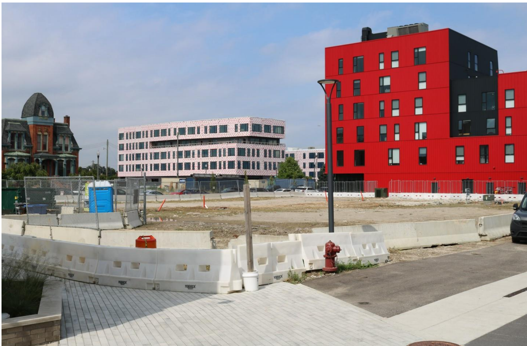
Staff photo of subject property, seen from vacated alley facing northeast. August 2022.
