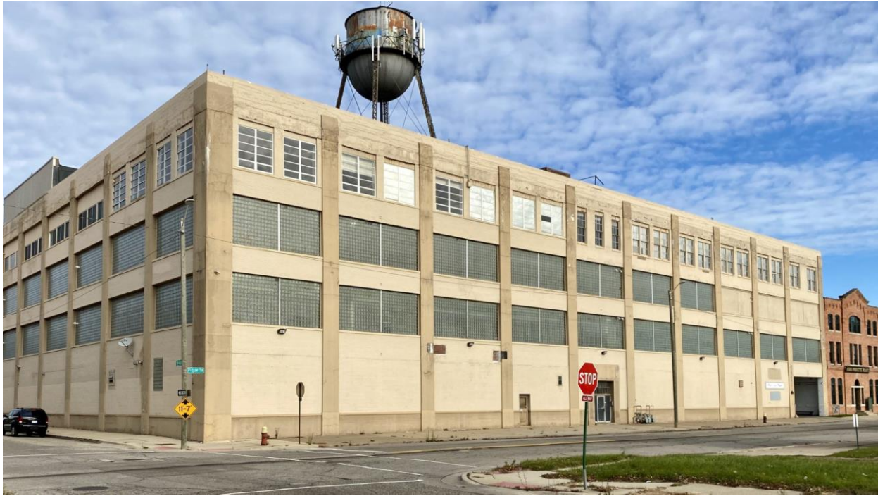
Site at the corner of Piquette Ave. and Beaubien St. in Milwaukee Junction. 10
