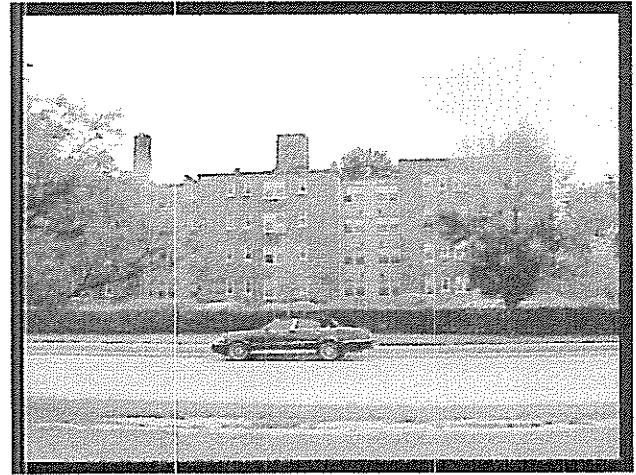
PICTURE D – APARTMENT TO EAST
