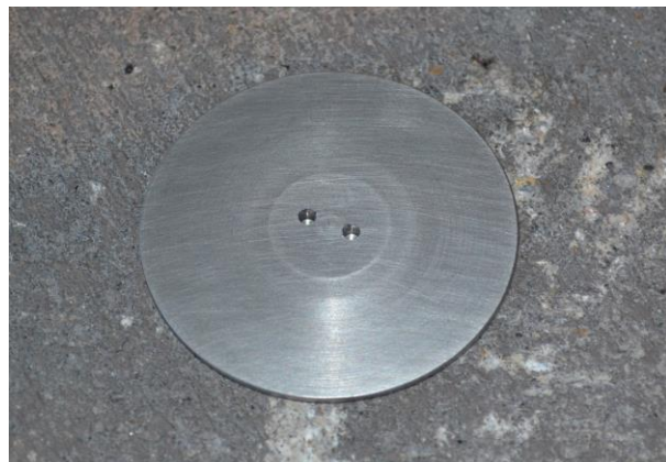
Figure 4. Secure Cover Installed
