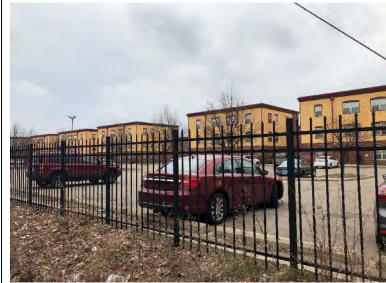
Photo 4. The north adjoining apartments
