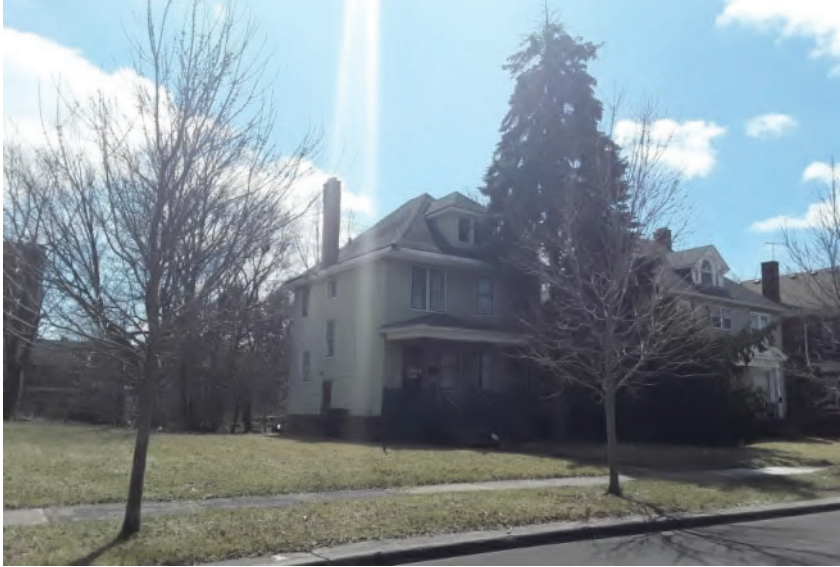
Southwest adjacent residential property – 1323 Seward Avenue (1912)
