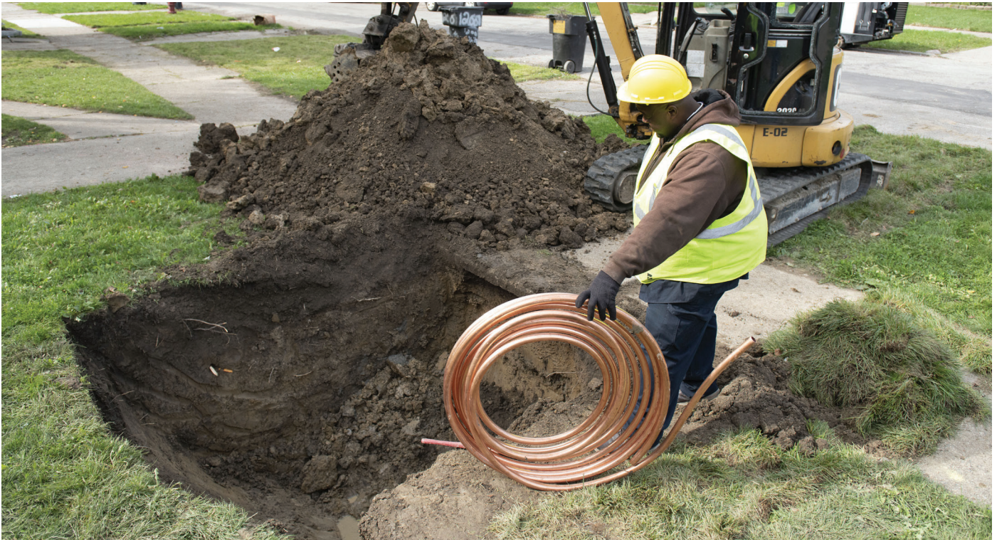
In 2018, DWSD began replacing lead service lines with copper, with owner/occupant permission, while on the same street replacing the water main.
