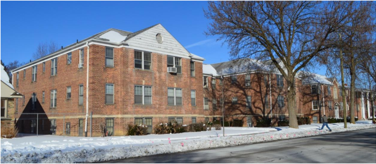
Photo 1 Looking northwest at 9730 (left) and 9710 (right) West Outer Drive, February 2021
