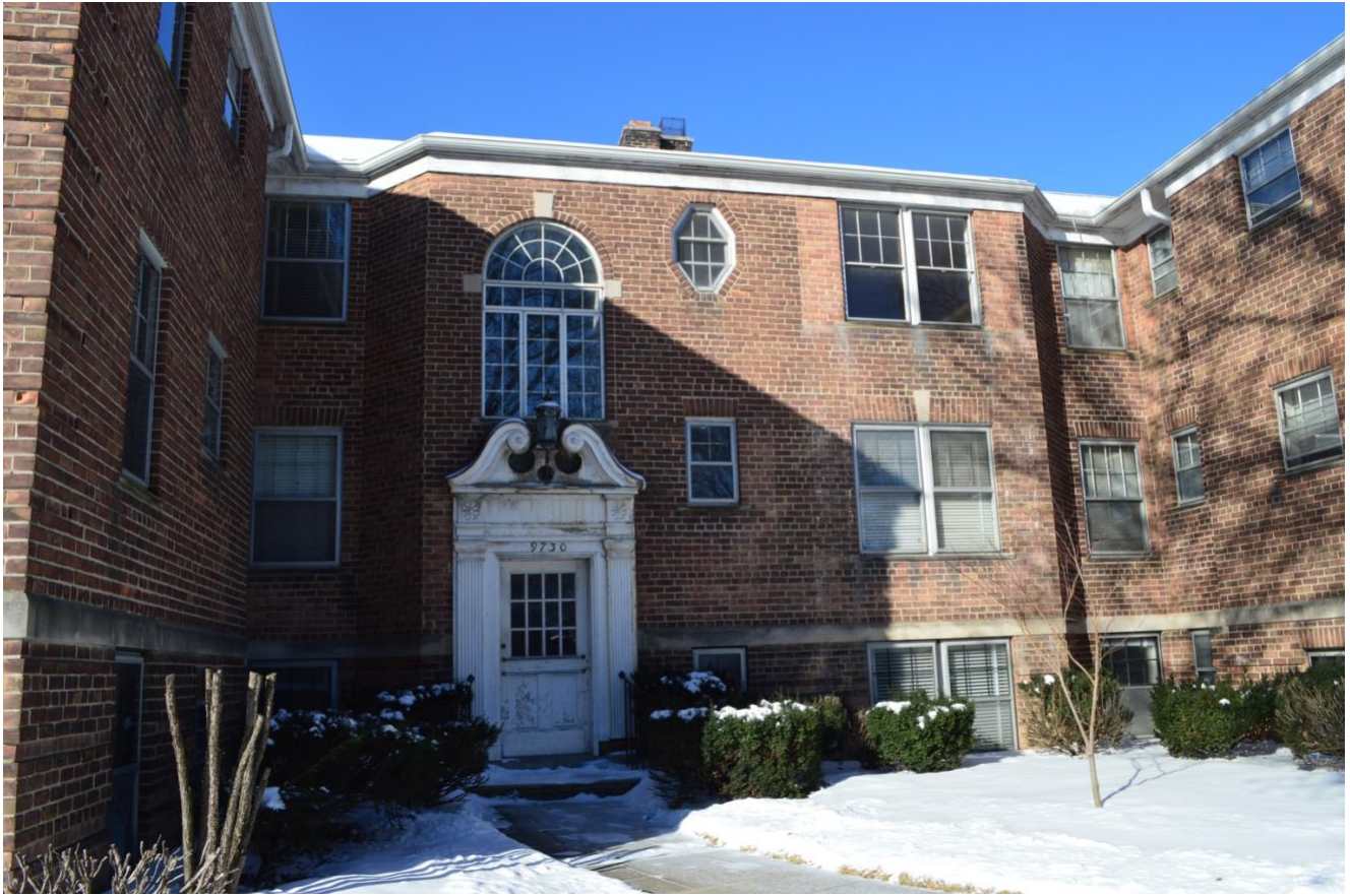
Photo 3 – Detail of entrance and courtyard of 9730, February 2021
