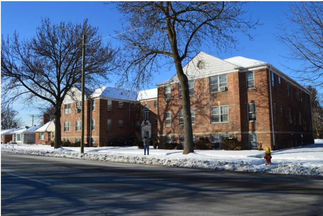
East façade and north elevation
