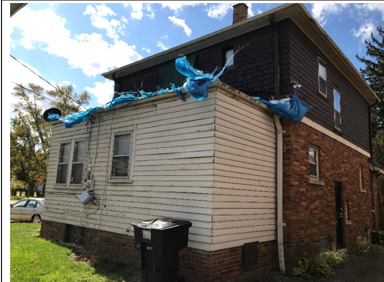
Photo 11. Side C of 15770 Minnock St.
