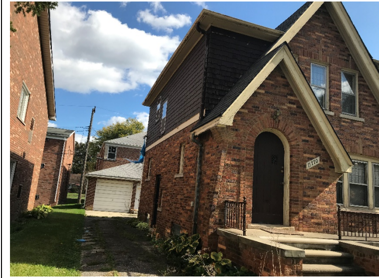
Photo 10. Side B of 15770 Minnock St.
