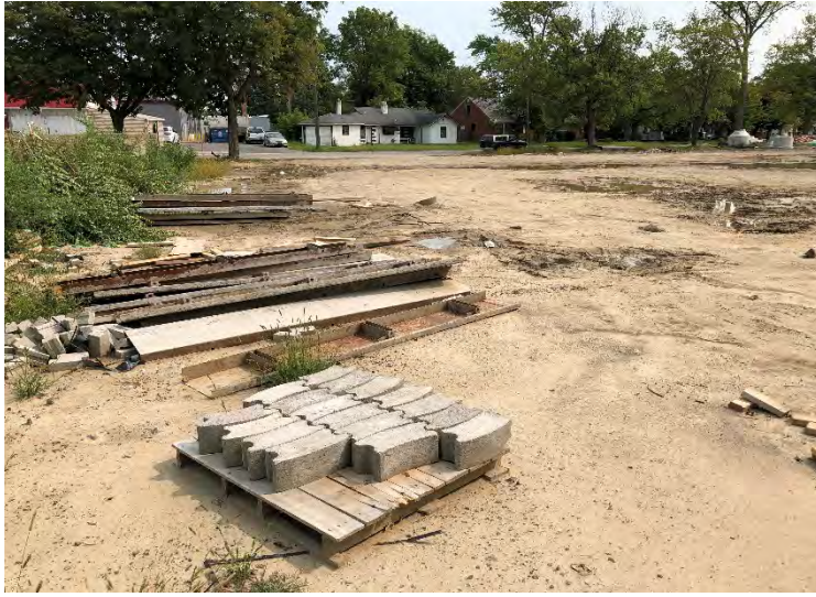
Photo 1. View of typical construction storage items on site
