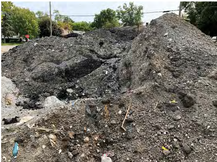
Photo 3. A closer view of the crushed asphalt pile
