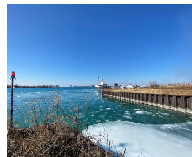
Entry channel and seawall
