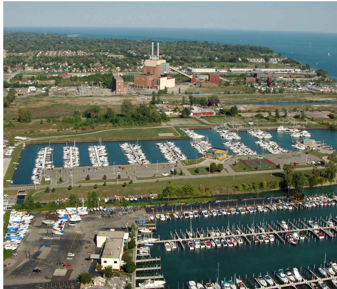
Aerial view of existing Engel Park and Reid Park along the Detroit River
