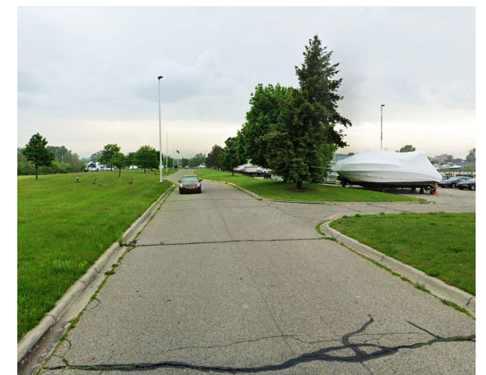
Riverside Marina's main drive lane has cracked pavement and lacks pedestrian infrastructure
