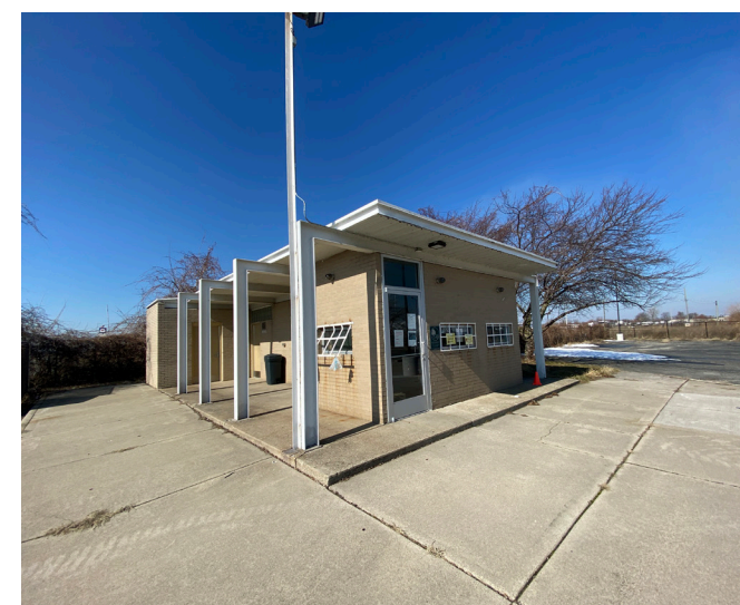
Office and public restrooms building
