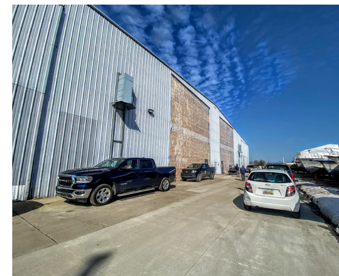
Temporary doors on the indoor storage building
