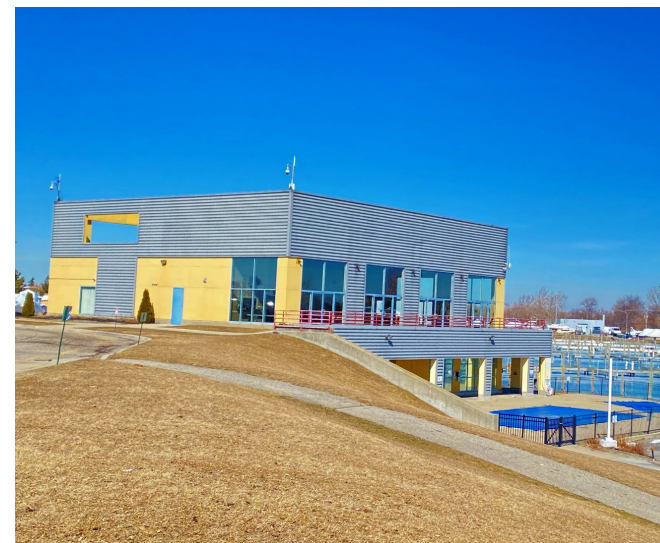
The Office/Clubhouse building is in need of upgrades
