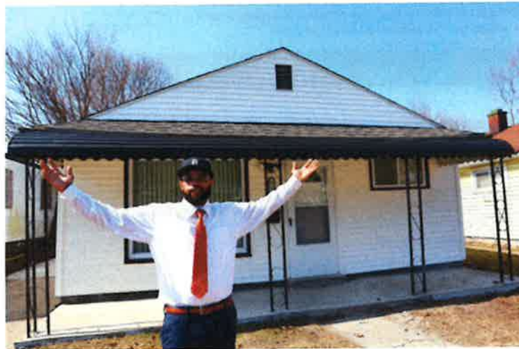
DLBA Success Story Buyer Melvin Walker outside his renovation on Alpine in District 6's Midwest neighborhood.
