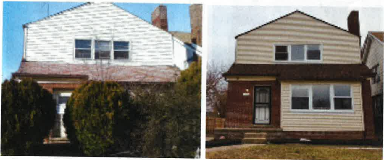
Before and After, renovated as a result of a NAP Abatement Agreement –Leslie, District 7
