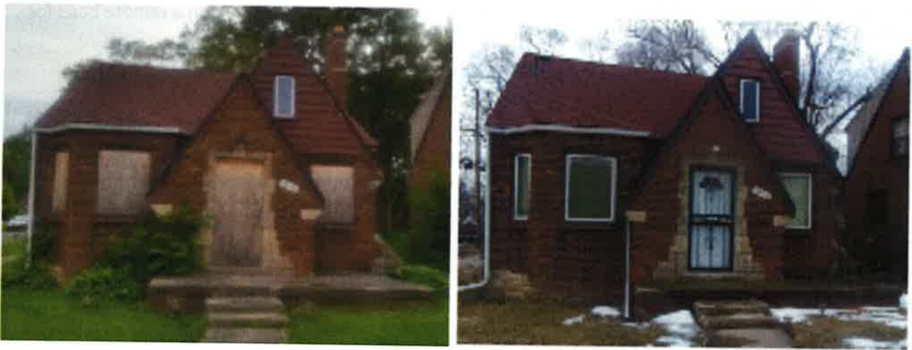
Before and After, renovated as a result of a NAP Abatement Agreement –Ferguson, District 1
