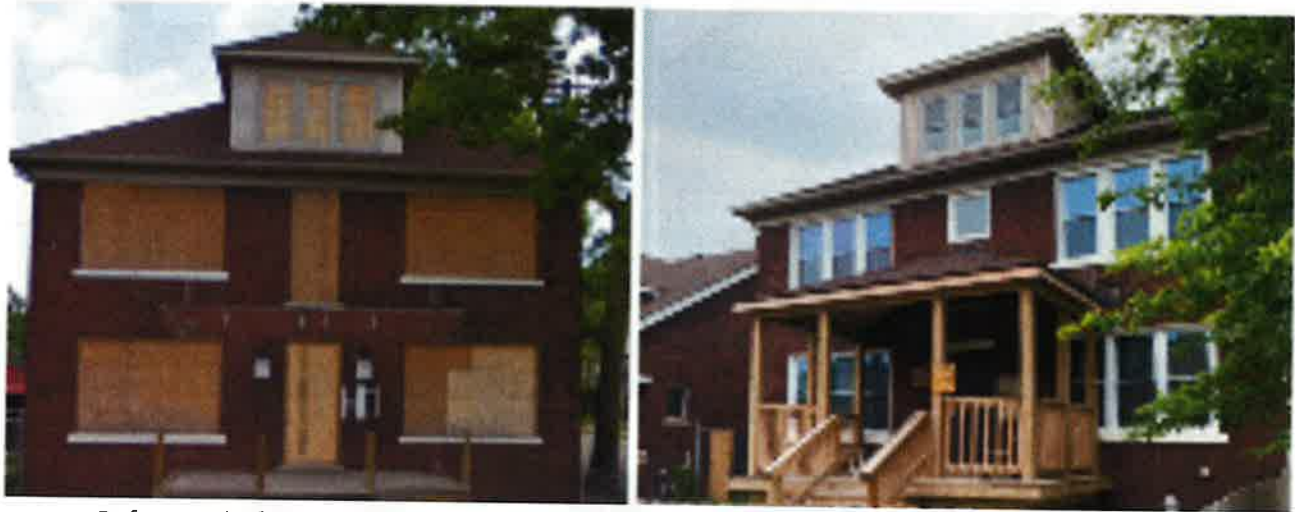
Before and After, renovated as a result of a NAP Abatement Agreement –Central, District 6
