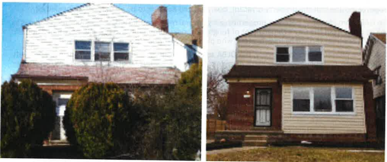
Before and After, renovated as a result of a NAP Abatement Agreement –Santa Rosa, District 2
