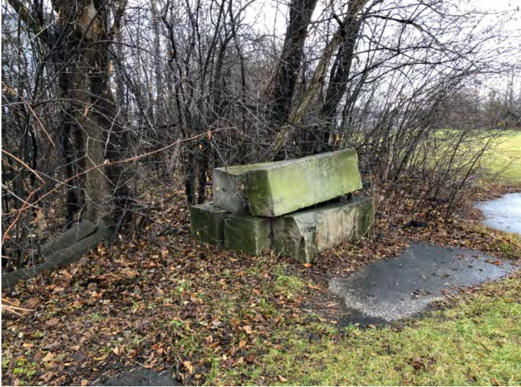
Photo 7. Masonry walls debris located to the northeast of the Subject Property
