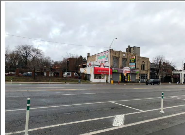
Photo 15. Northeast adjoining properties located on 7869 and 7875 E Jefferson
