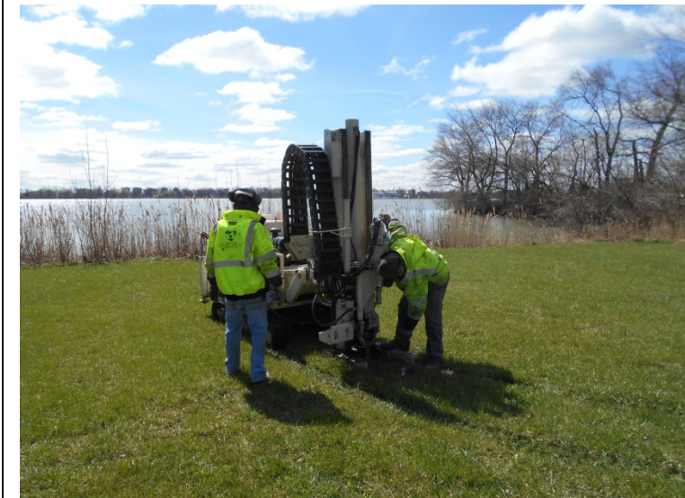
Photo 6. Advancement of soil boring SB-5
