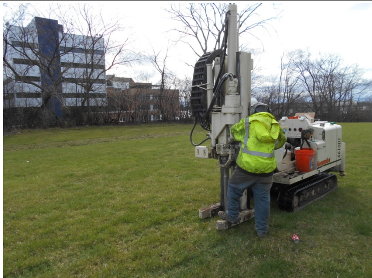
Photo 2. Advancement of soil boring SB-2
