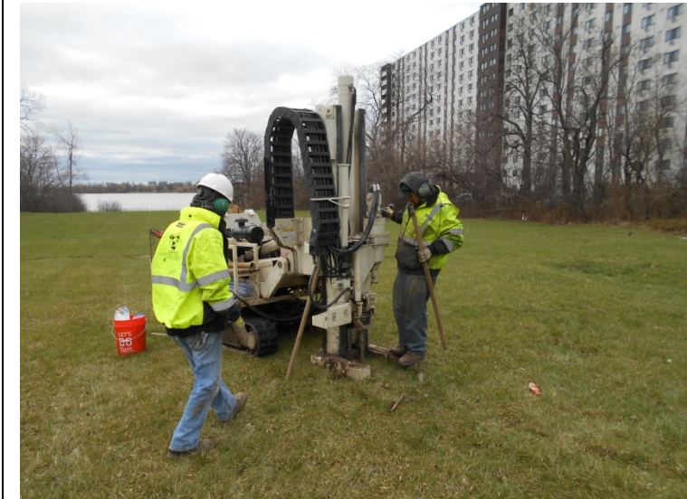
Photo 1. Advancement of soil boring SB-1
