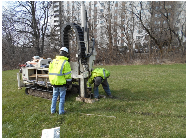
Photo 3. Advancement of soil boring SB-3
