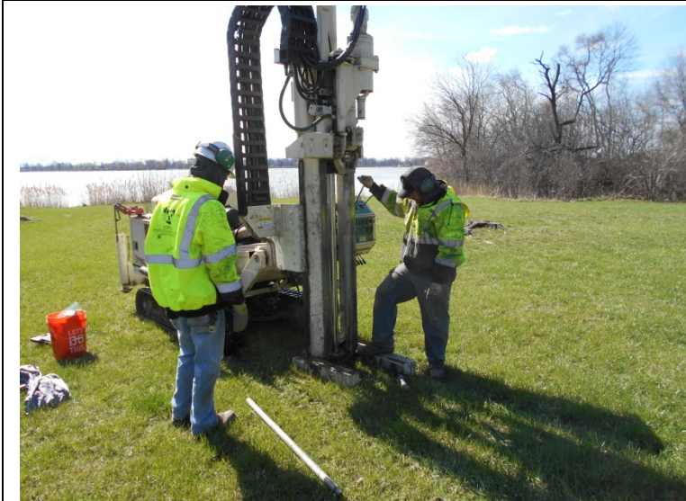
Photo 5. Advancement of soil boring SB-4
