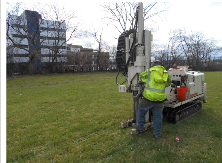
Photo 2. Advancement of soil boring SB-2
