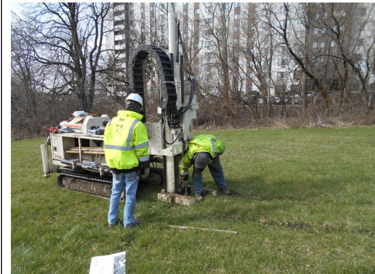
Photo 3. Advancement of soil boring SB-3
