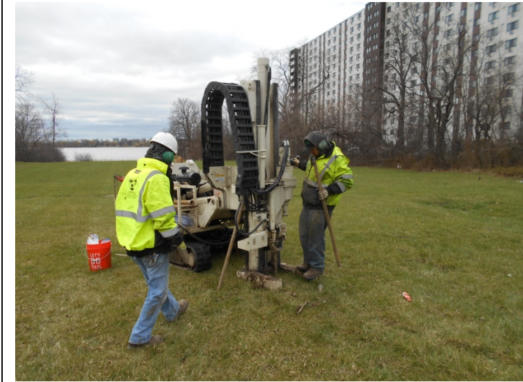
Photo 1. Advancement of soil boring SB-1
