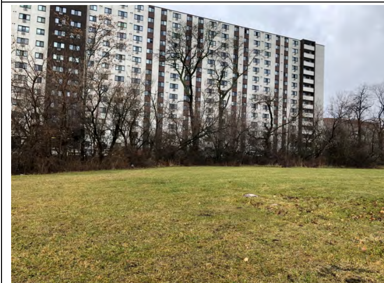
Photo 5. The west view of the Subject Property
