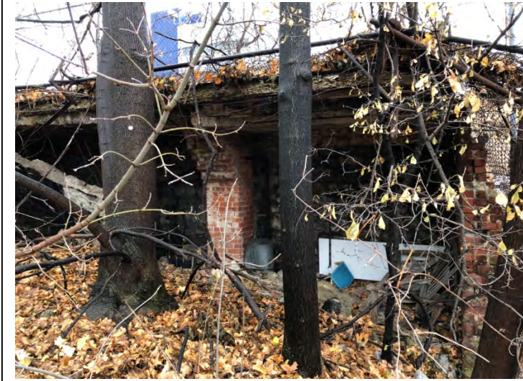
Photo 10. Old building remains located to the southeast of the Subject Property
