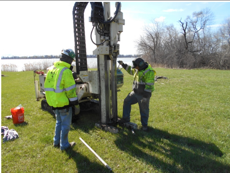
Photo 5. Advancement of soil boring SB-4
