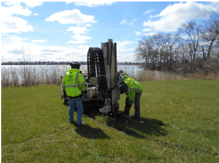
Photo 6. Advancement of soil boring SB-5
