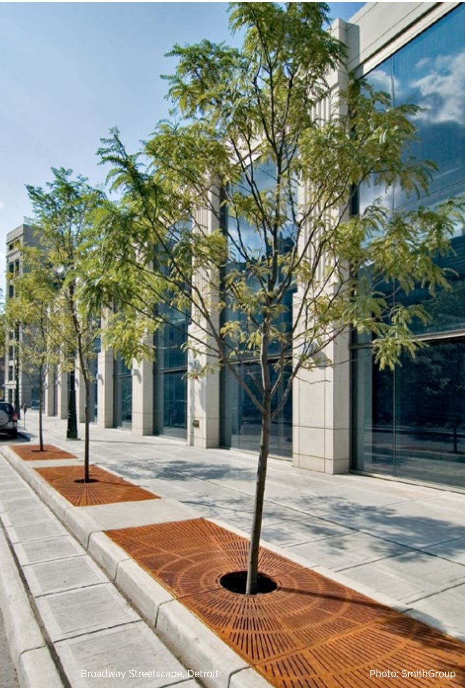
Ironsmith 'ADA' 4ft. x 12ft. 12" x12" opening Cast Ductile Iron with Baked on Oil-finish Load Class C ADA compliant
