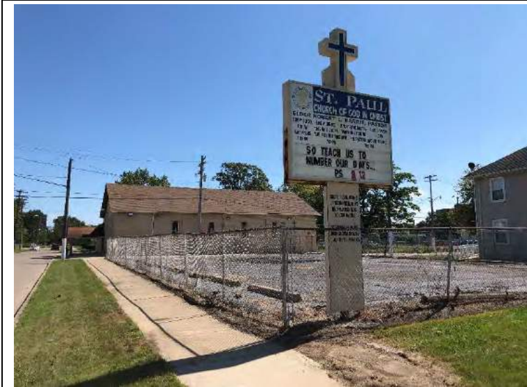
Photo 14. The adjoining church on Sheridan and Agnes
