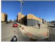
② EXISTING CORNER AT E. JEFFERSON AVE AND HOLCOMB ST
