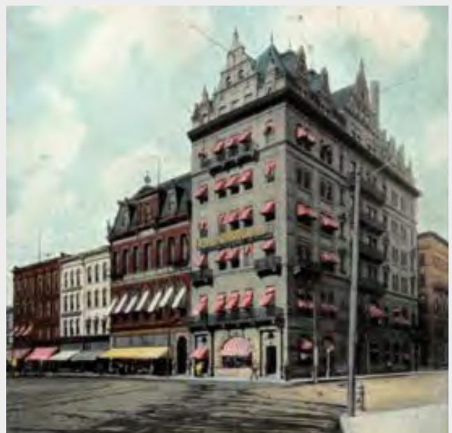
The site once hosted the 7-story St. Claire hotel—an apartment building that was demolished in 1934.
