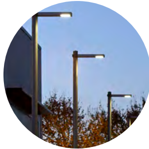
Street Lighting (20' H)
