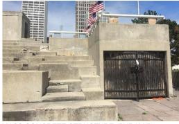
MASS CONCRETE STRUCTURE (PYRAMID)
