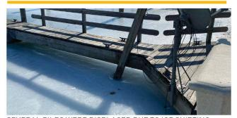
SEVERAL PILES WERE DISPLACED DUE TO ICE SHIFTING
