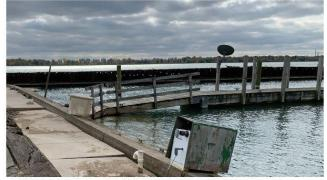
SEVERAL SPUDS AND ANCHOR POINTS WERE OUT OF ALIGNMENT OR IN A LOCKED POSITION
