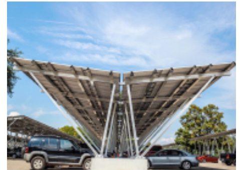
Figure 13: Solar parking lot bays in East Lansing MI (MSU)
