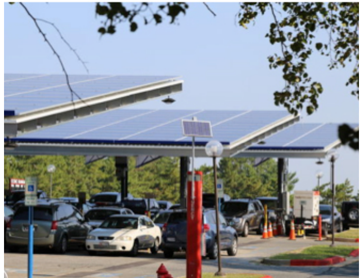
Figure 14: Community solar “canopy” over parking lot in BGEC Community Pilot Site 19
