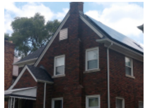
Figure 10: Single family rooftop array in Detroit (Cherrylawn-Northwest)
