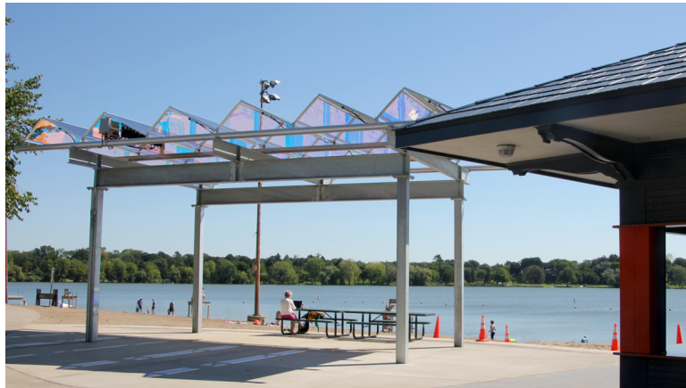
Solar pavilion in a Minneapolis park 7
