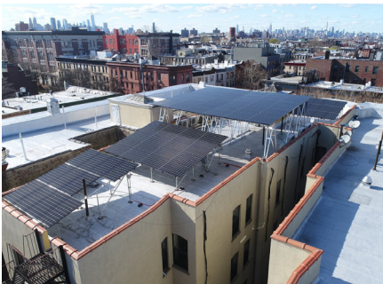
Brooklyn Solar Work's canopy installation on the Crown Heights co-op 9
