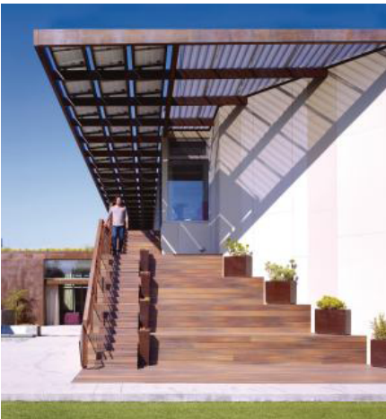
Integrated solar awning on the Yin-Yang House in Venice, California 2
