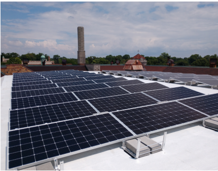
Rectilinear rooftop array on Gesu Catholic School 1
