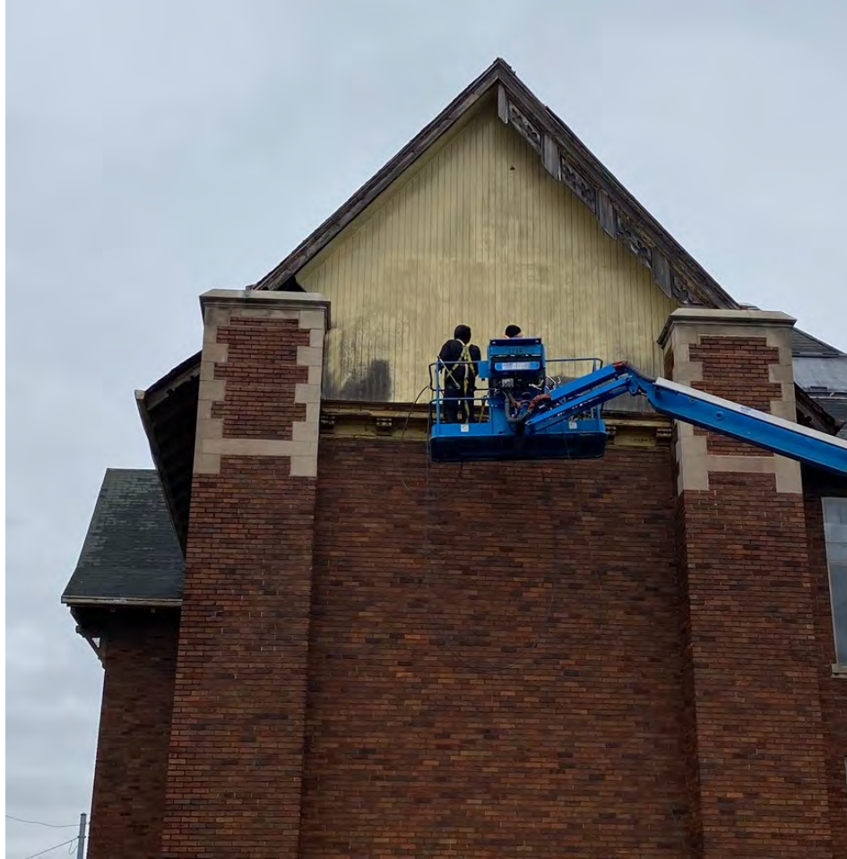
ONGOING REPAIRS & MAINTENANCE TO PRESERVE BUILDINGS
