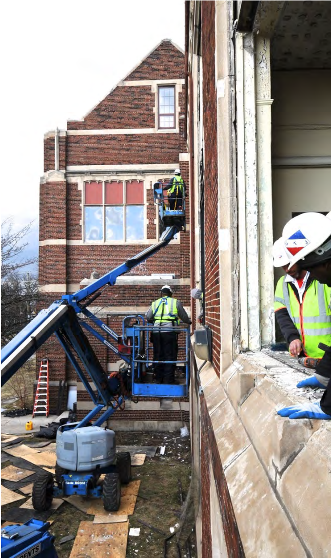
CROSMAN + HUTCHINS SCHOOLS : WINDOWS CLEAR BOARDED + PERIMETER SECURED
