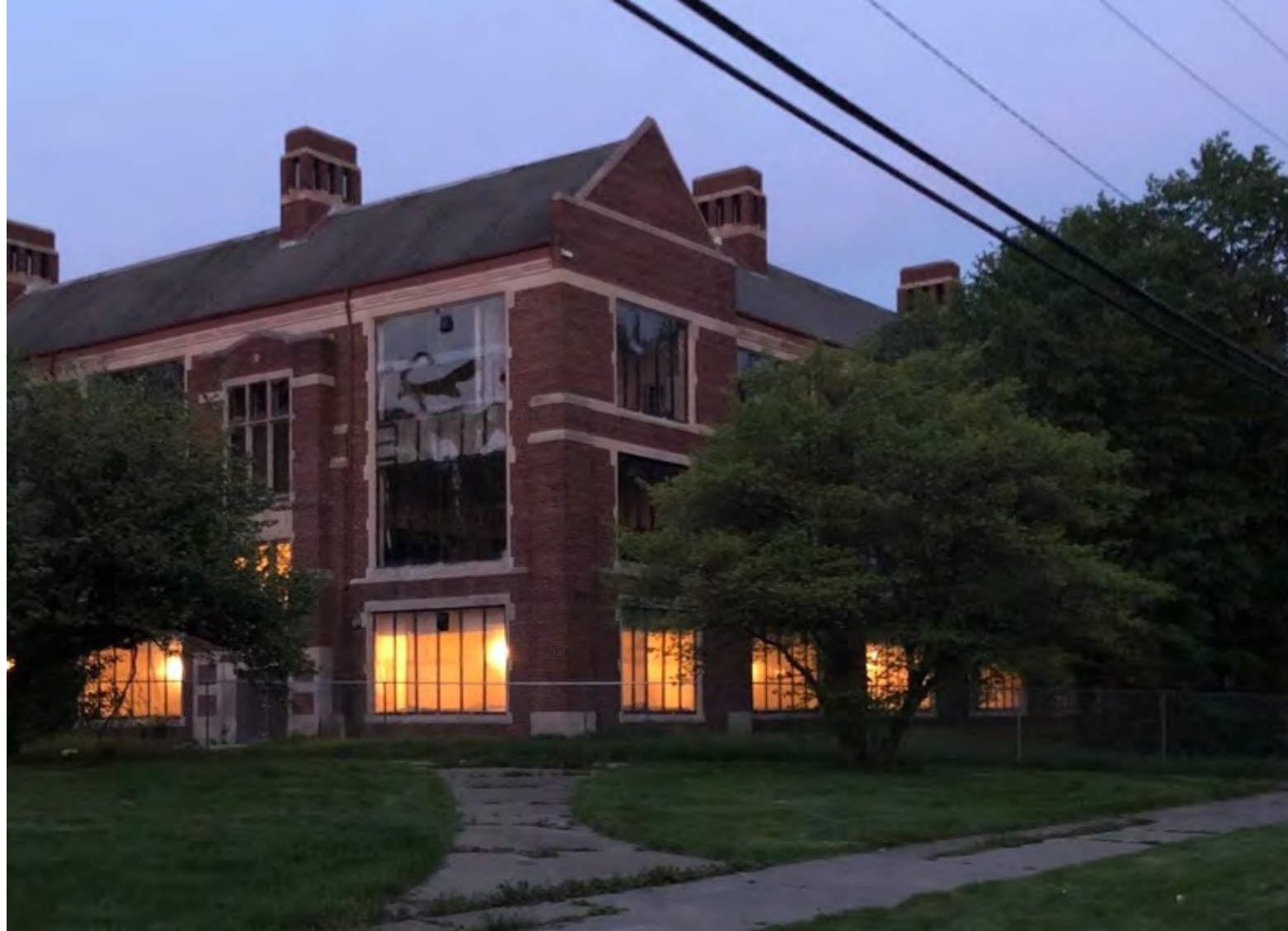
TEMPORARY SAFETY LIGHTING
