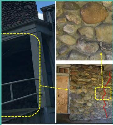
portion of the fieldstone chimney and vertically oriented crack
