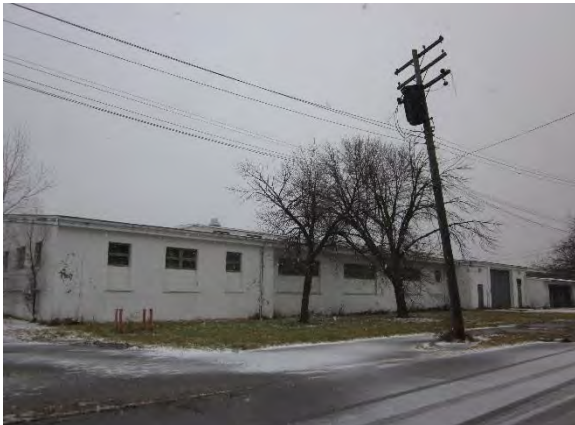
Barn/Storage (Photo Taken on January 12, 2018)
