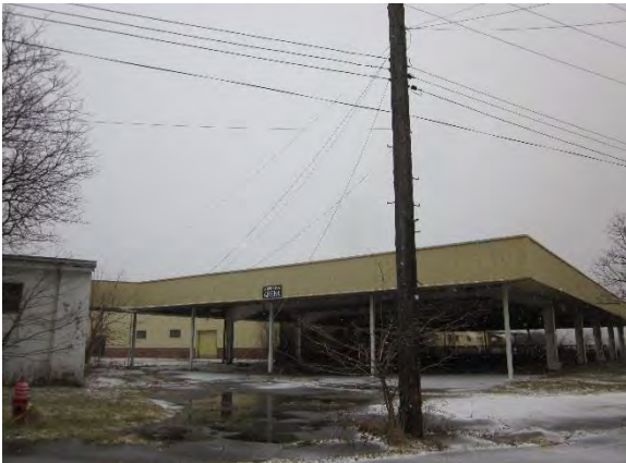
Shelter (Photo Taken on January 12, 2018)
