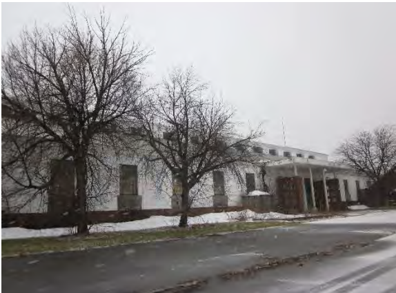
Side of Agriculture Building (Photo Taken on January 12, 2018)
