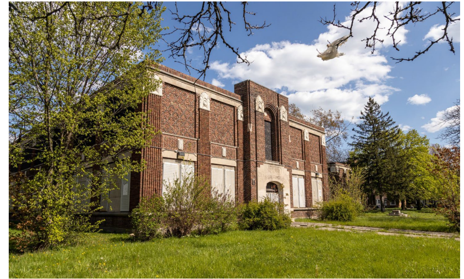
Former Burbank Elementary
