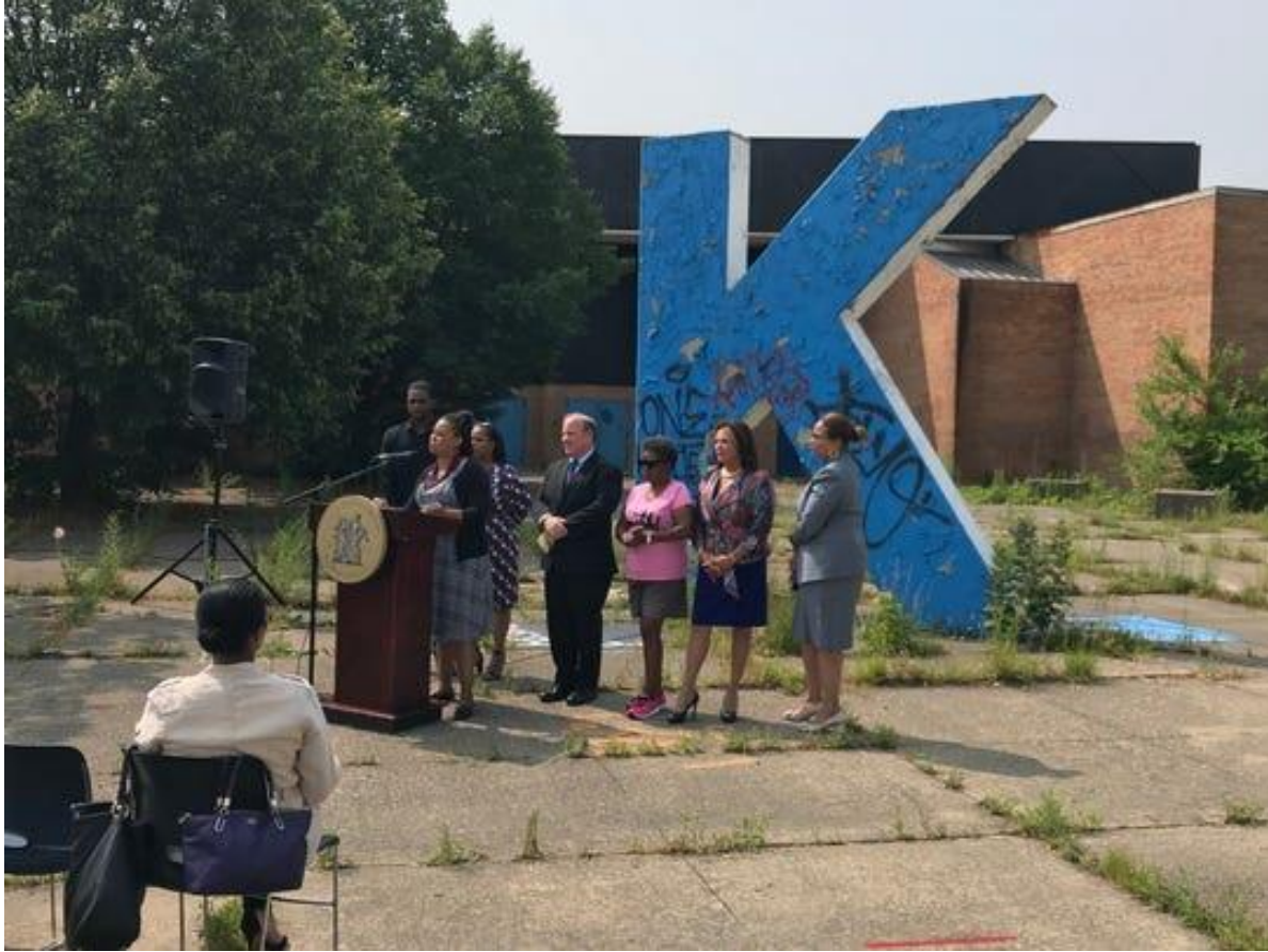
The only piece of the school expected to survive construction is the large blue Kettering (High School) "K" on the site. 8
