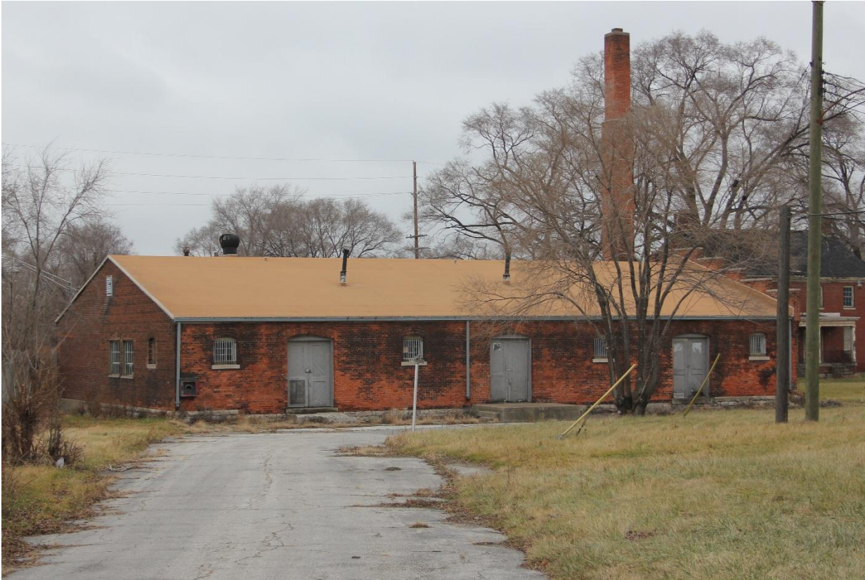
Front (south) facade, April 2019
