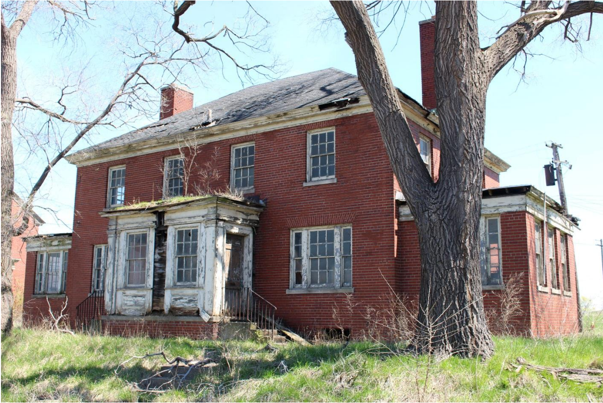
Front (northwest) facade, April 2019
