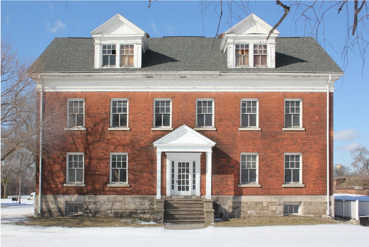
Front (south) facade, April 2019
