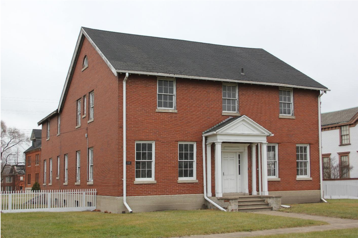
Front (south) facade, April 2019
