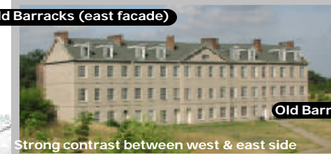
Old Barracks (east facade)
