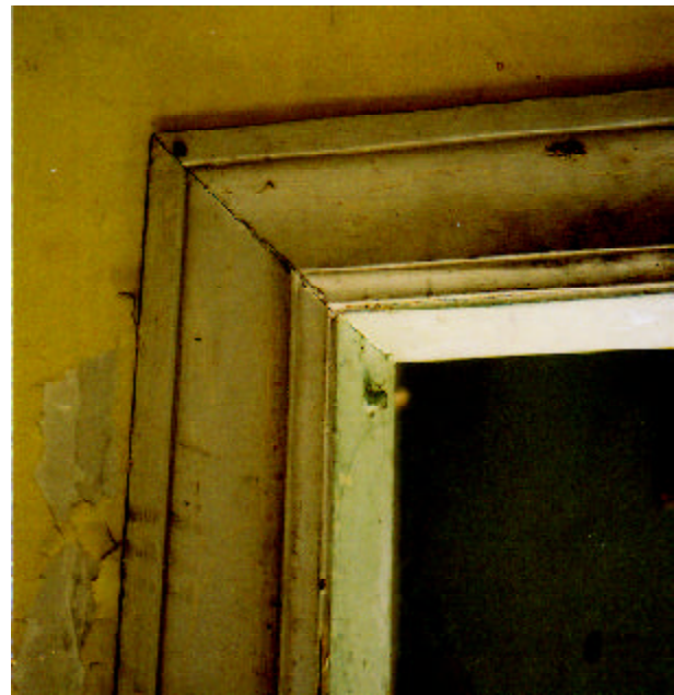
1930's Remodeled Door Casing
