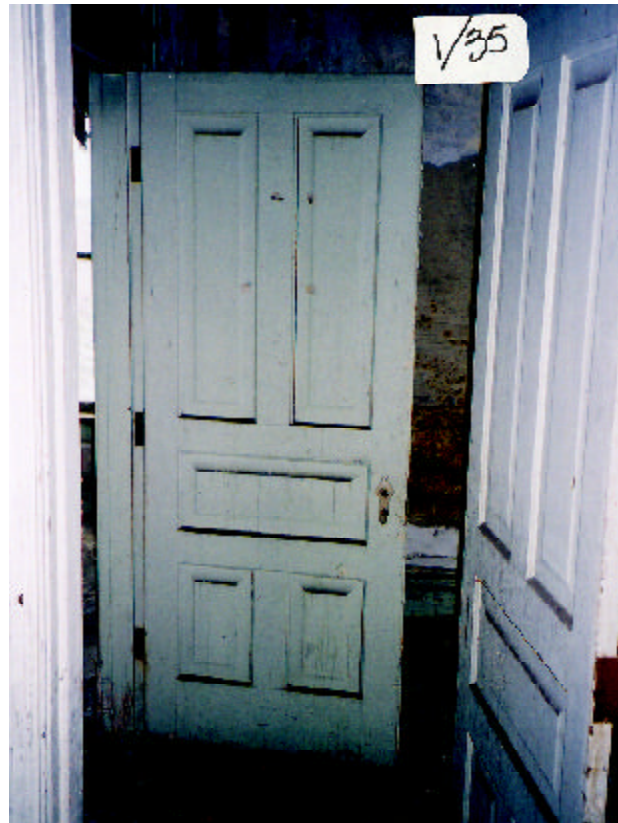
Intact Five Paneled Door (hardware missing)
