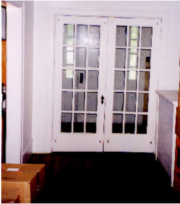
Intact 15 Lite Glazed Doors
