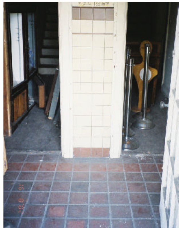
1930's Vestibule Quarry Tile Floor and Ceramic Tile Wainscot
