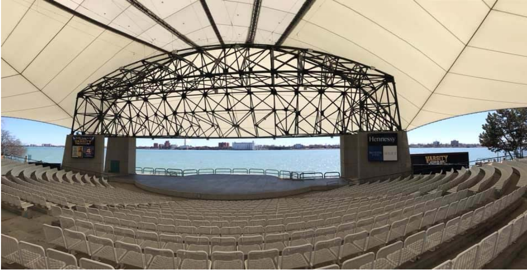
(J) Stage with added wings-note stage house overhead for tensile roof base
