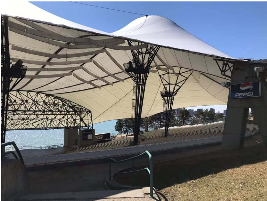
(I) Tensile Roof over Fixed Seating-Looking south
