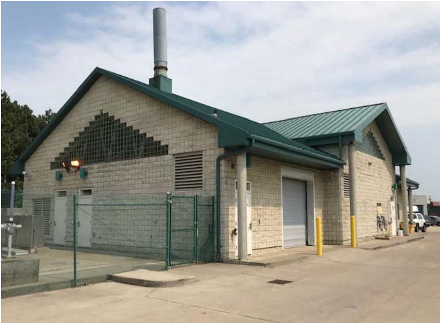
(L) Water & Sewage Department Building - looking southeast
