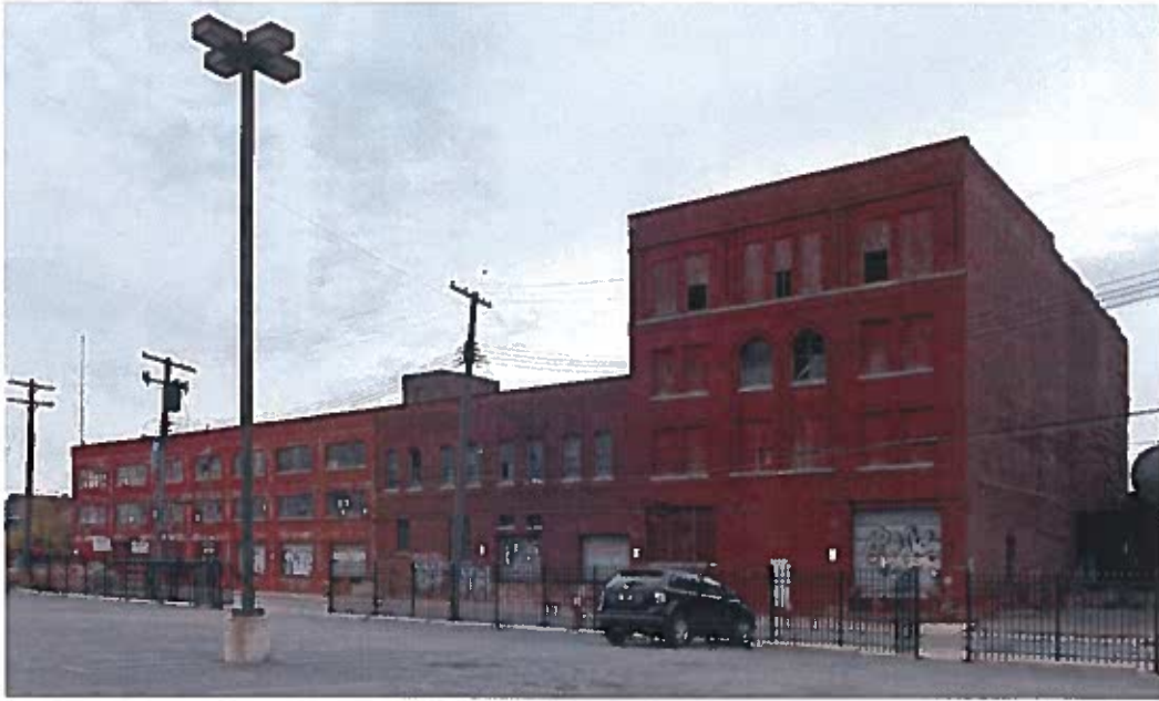
The Stone Soap building in Detroit's east riverfront district was constructed in phases starting in 1907 and ending with the final structure in 1927-29. 8
