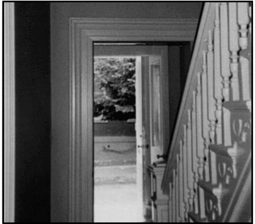
Figure 18.3 Historic Property Where the Interior Woodwork and Staircase Were Wet Sanded and Recoated With Three Layers of Encapsulant To Preserve the Carved Profiles.
