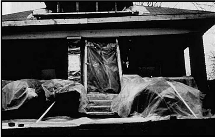
Figure 8.3b Prepare the Worksite With Plastic Sheetting (exterior).
