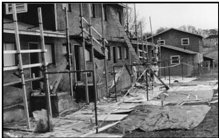
Figure 12.6 Exterior Siding Removal and Replacement.
