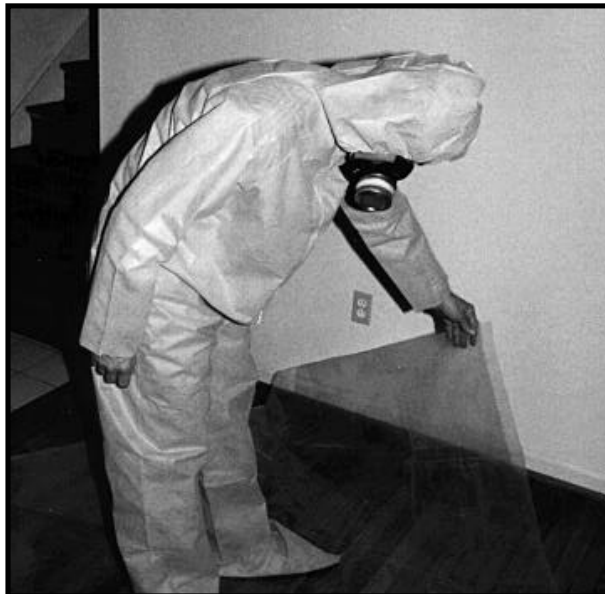
Figure 14.8a Pick Up Corners of Plastic Sheeting.
