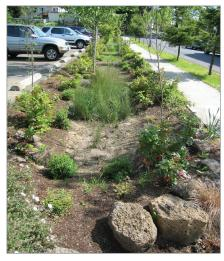
The stormwater in this parking lot flows to the outside edge where a vegetated bioretention practice was installed to manage the water before it leaves the property
