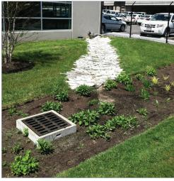
Stormwater from the building's downspouts is directed into this bioretention practice
