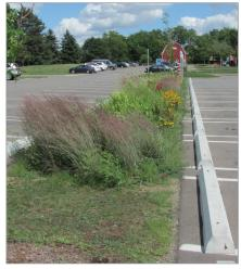
An existing parking lot in Southfield, Michigan, was restriped and a section of pavement at the low point was removed and planted for stormwater management
