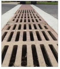
An example of a trench drain installed to capture runoff prior to entering the catch basin connected to DWSD's sewer system
