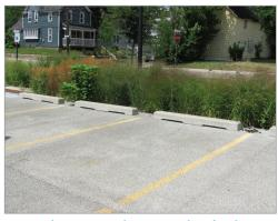
Linear bioretention along outer edge of parking area captures the runoff
