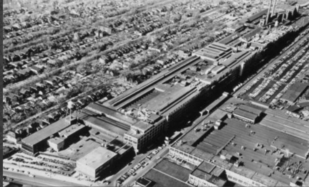
1954 Mack Avenue Stamping Plant (formerly Briggs Mack Avenue)
