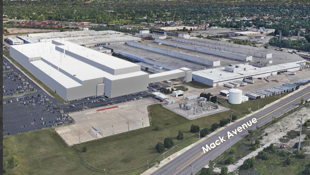
Future Mack Avenue Assembly Plant
