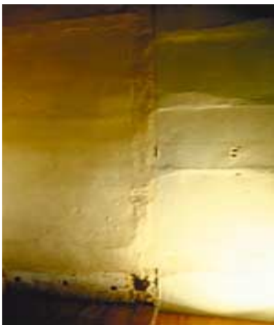
Raking light is used to show irregularities on flat surfaces. Patches, repairs, and alterations can then be mapped by the shadows or ghosts they cast. Photo: Travis C. McDonald, Jr.
