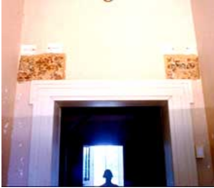
Destructive investigation can be limited to small areas where evidence can be predicted, such as walls being re-built in a different location. Photo: Travis C. McDonald, Jr.
