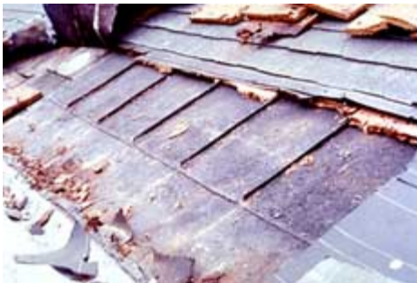
In many cases, new materials or coverings are placed directly over existing exterior features, preserving the original materials underneath. Here, the removal of a modern shingle roof and its underlayment revealed an historic standing seam metal roof. Photo: Courtesy, Phillips and Opperman, P.A.
