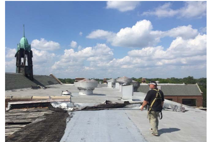
HUTCHINS SCHOOL: • ROOF FIXED, WINDOWS CLEAR BOARDED, PERIMETER SECURED
