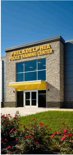
^PHILADELPHIA POLICE TRAINING FACILITY
