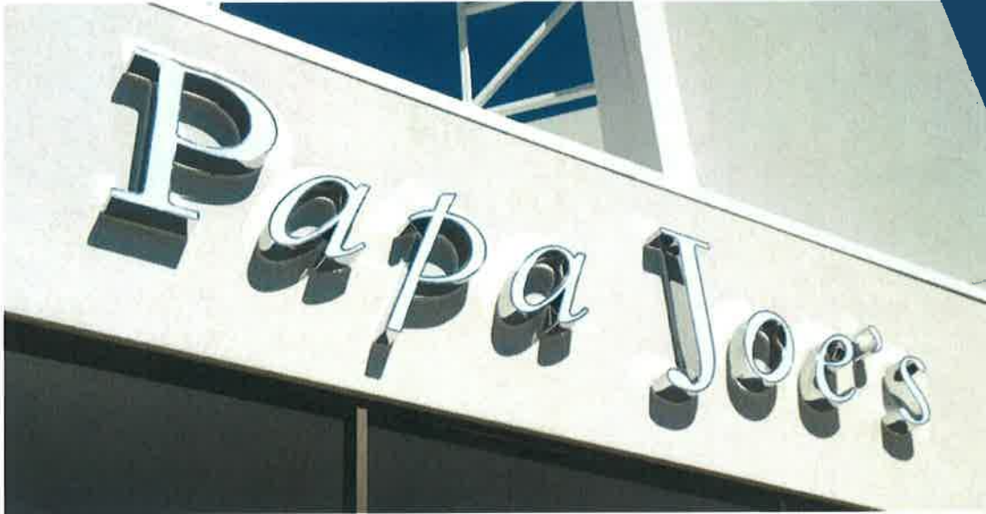
SIGN DURING THE DAY WHITE PLEXIGLASS FACES WITH POLISHED STAINLESS STEEL RETURNS
