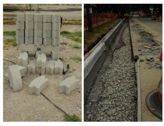
Figure 21 Keeler Street Permeable Paver Construction Photos
