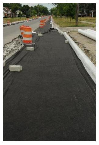
Figure 20 Artesian Street Porous Asphalt Construction
