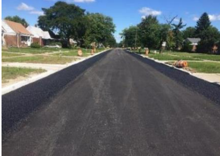
Figure 28 Artesian Street Porous Asphalt
