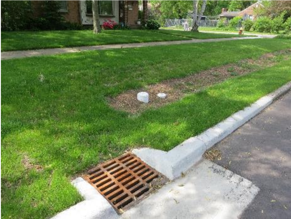
Figure 32 Tireman Phase I Bioswale
