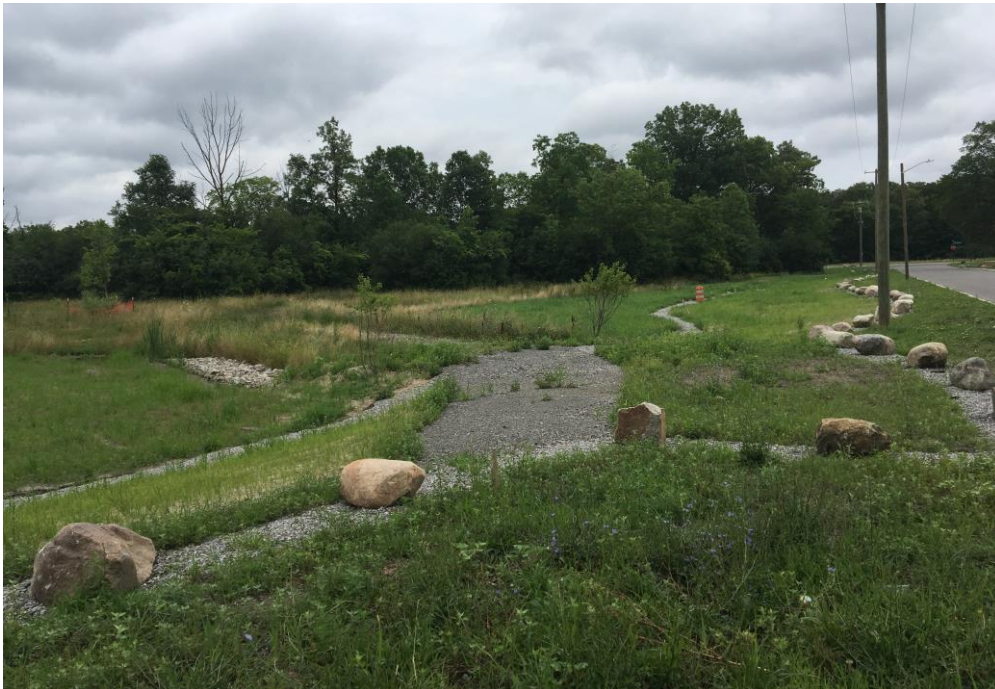
Figure 31 Tireman Avenue Bioswale - Phase II (North) at Substantial Completion
