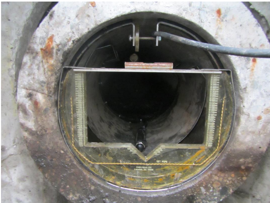
Figure 36 Installation of Compound Weir Prior to Beginning the Second Monitoring Period
