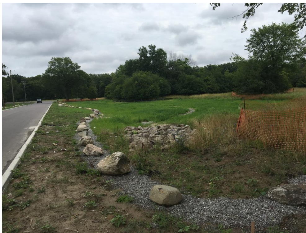
Figure 33 Tireman Avenue Bioswale - Phase II (South) at Substantial Completion
