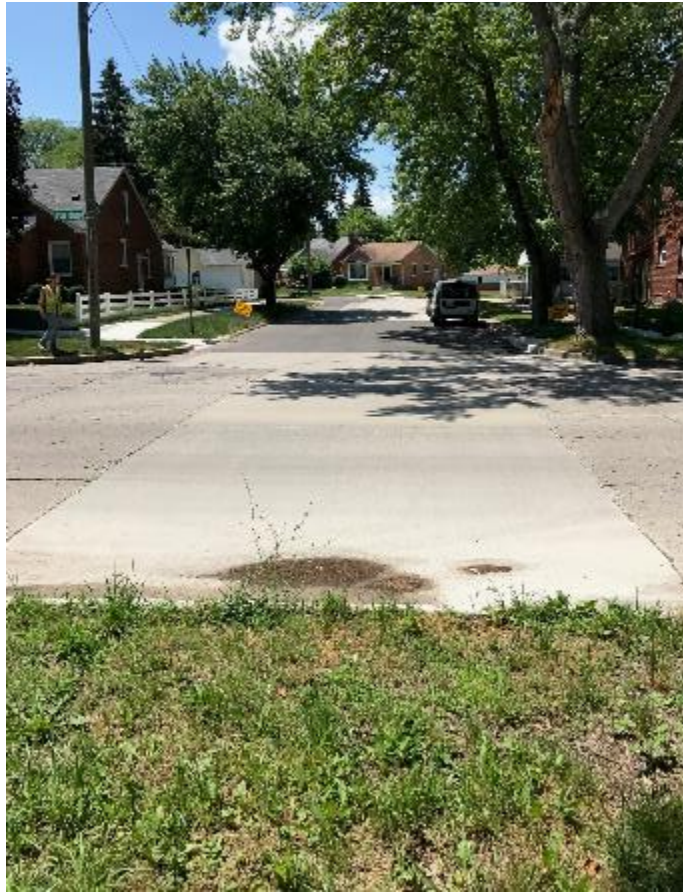
Figure 30 Road Restoration for Constance Storm Sewer
