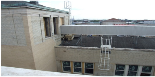
Main Library Roof Project Before Pictures
