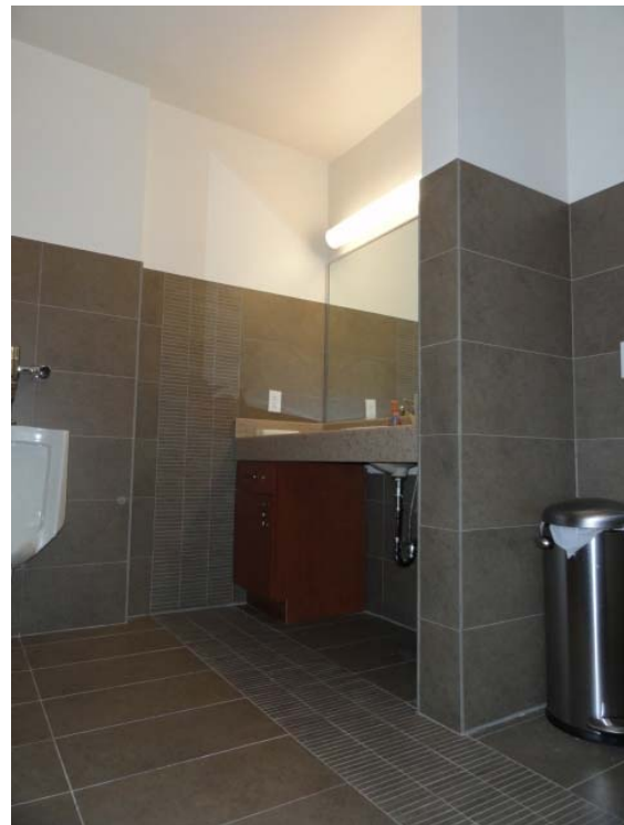
Fort Wayne - Building 112 - New restroom 2012
