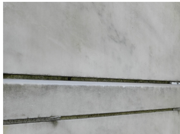
Main Library Eastwing tuckpointing
